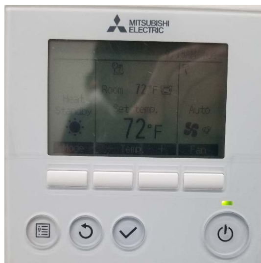
Figure 2. Heat pump thermostats in the front office were set to heat in the front office and in the conference room. This unnecessarily uses electricity when sites are closed and generally unoccupied.
