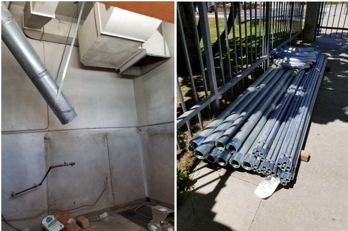
Figure 8. HVAC construction occurring at Webster Elementary
