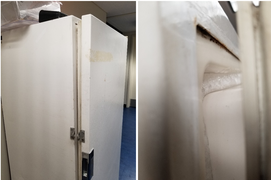
Figure 6. Freezer in the staff lounge was left plugged in, but the door was slightly open and frozen. This will need to be unplugged and slowly defrosted to be cleaned out. It is recommended to keep this unit unplugged throughout the remainder of the closure.
